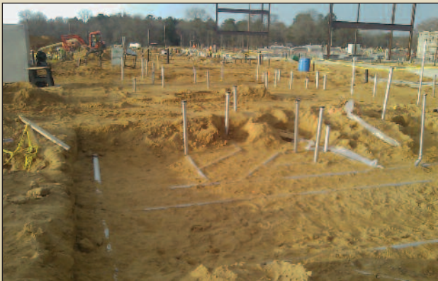
A Josam Push-Fit installation at New Cherry Hospital in Goldsboro, N.C.
