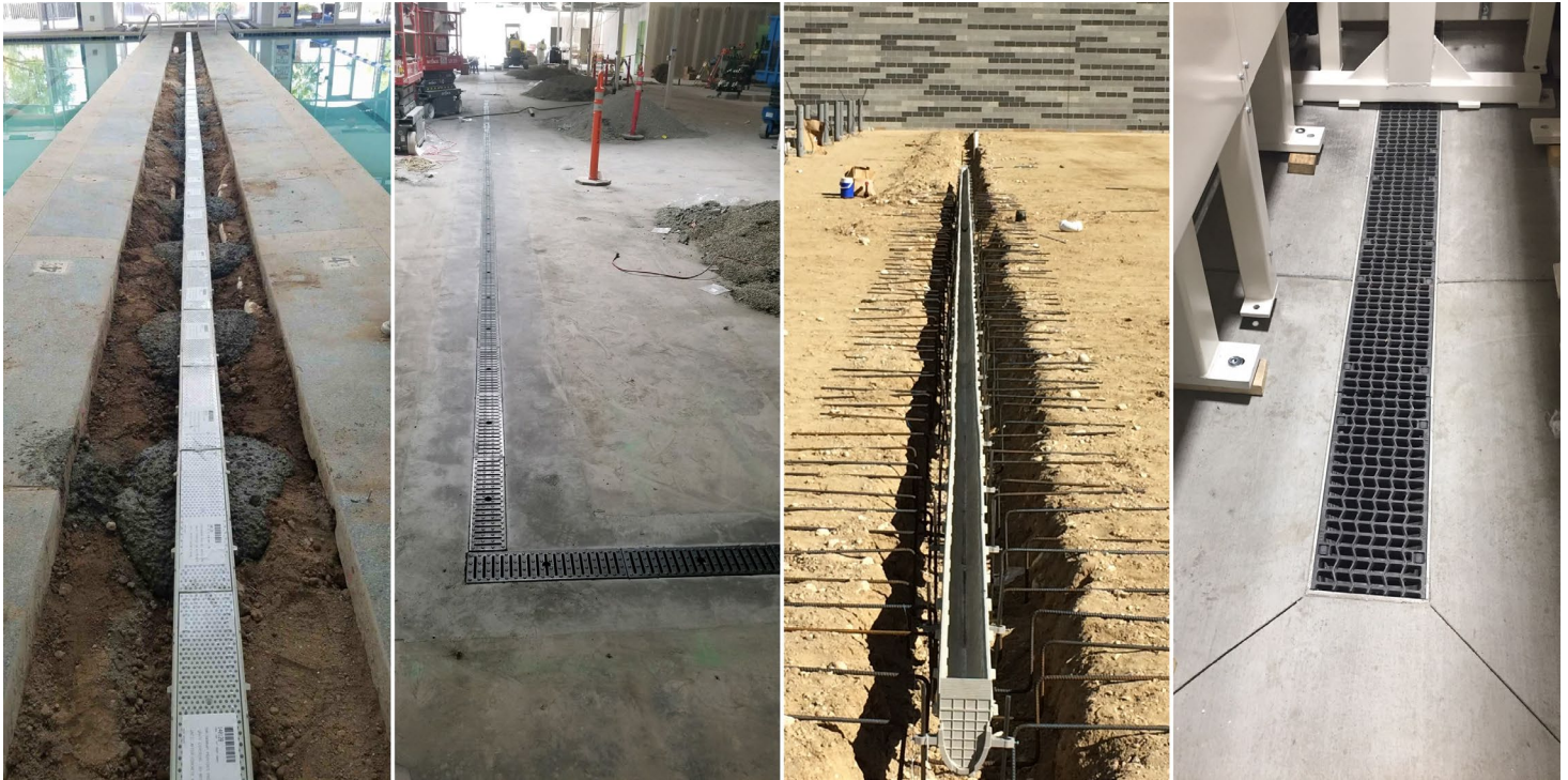
Installation images of Josam's PRO-PLUS™ Trench Drain System
