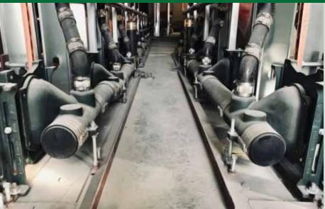
Josam Company recently introduced the CHASE SAVER III fitting. This fitting features a 3" pipe size that was engineered for project installations that require chase space savings. It's the perfect option for designs with narrow walls and more interior space.
