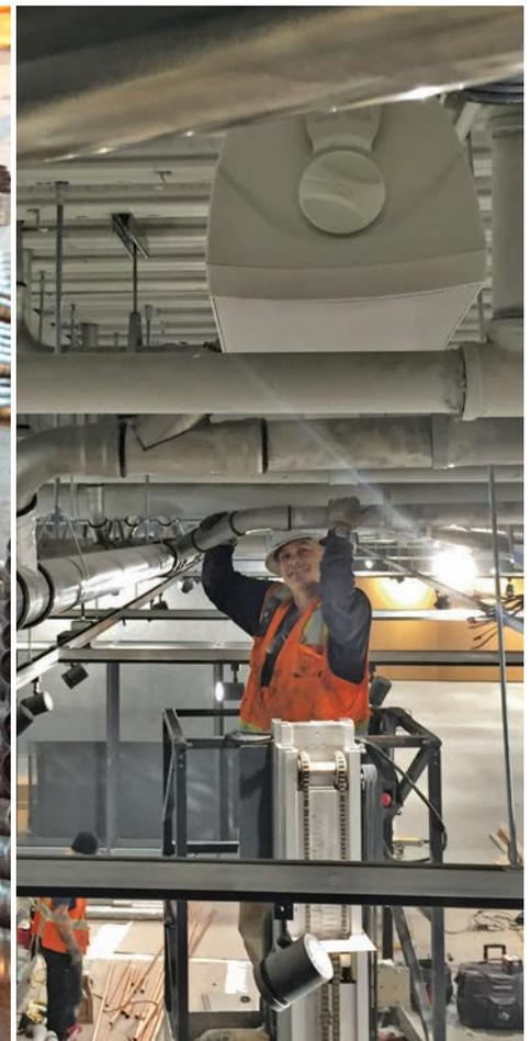
**Right:** All Area Plumbing specified Josam stainless steel waste and vent piping systems for a restaurant because the product could stand up to abuse by employees and corrosive chemicals. **Far Right:** Josam's Push-Fit joining system made installation easy for All Area Plumbing, even when combined with locking collars to provide extra durability.
